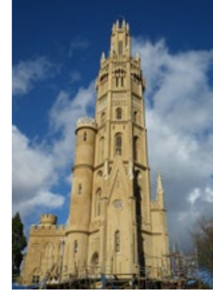
↘ Hadlow Tower, United Kingdom Identical restoration
