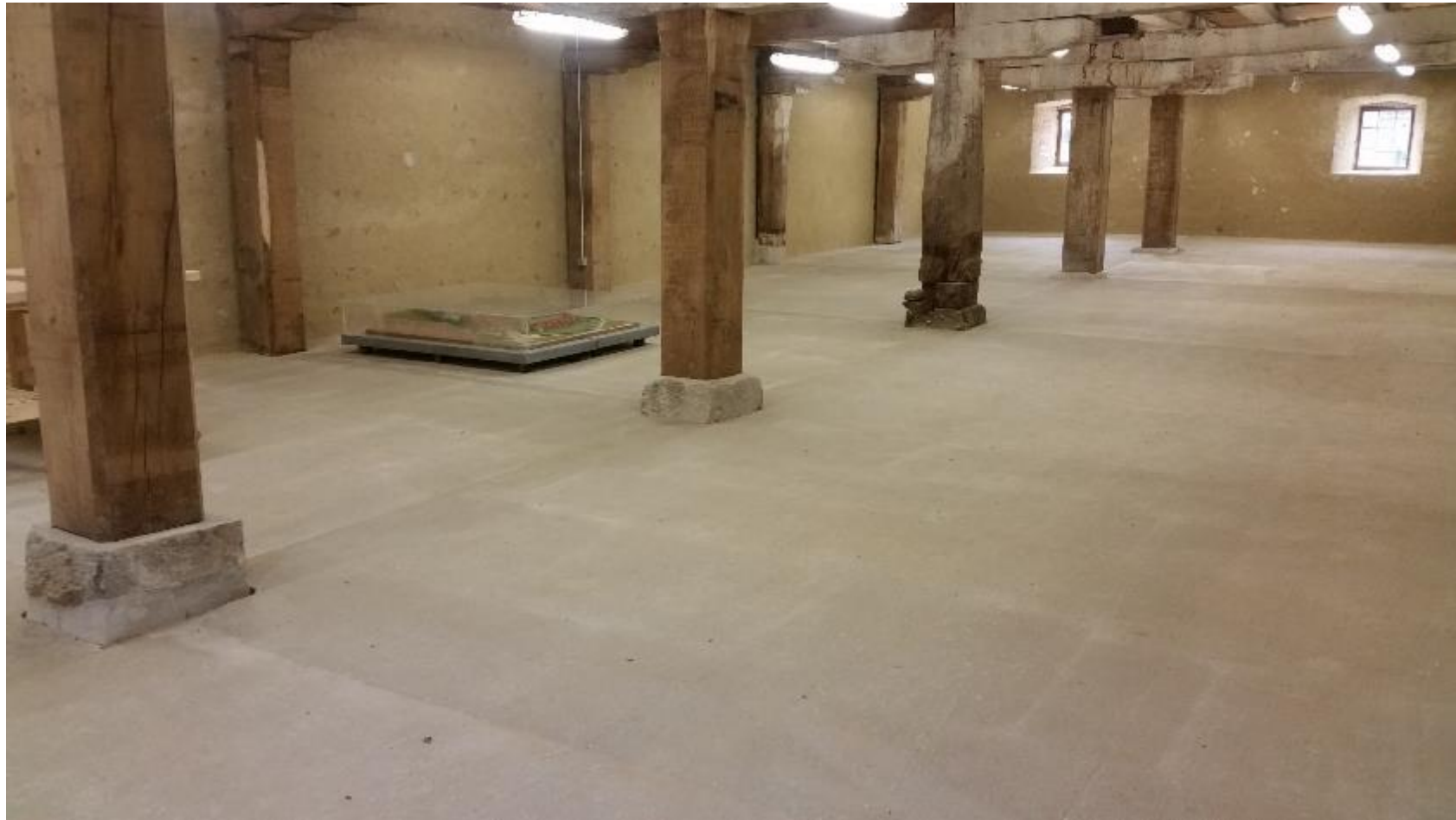
Lime / Prompt concrete floor
