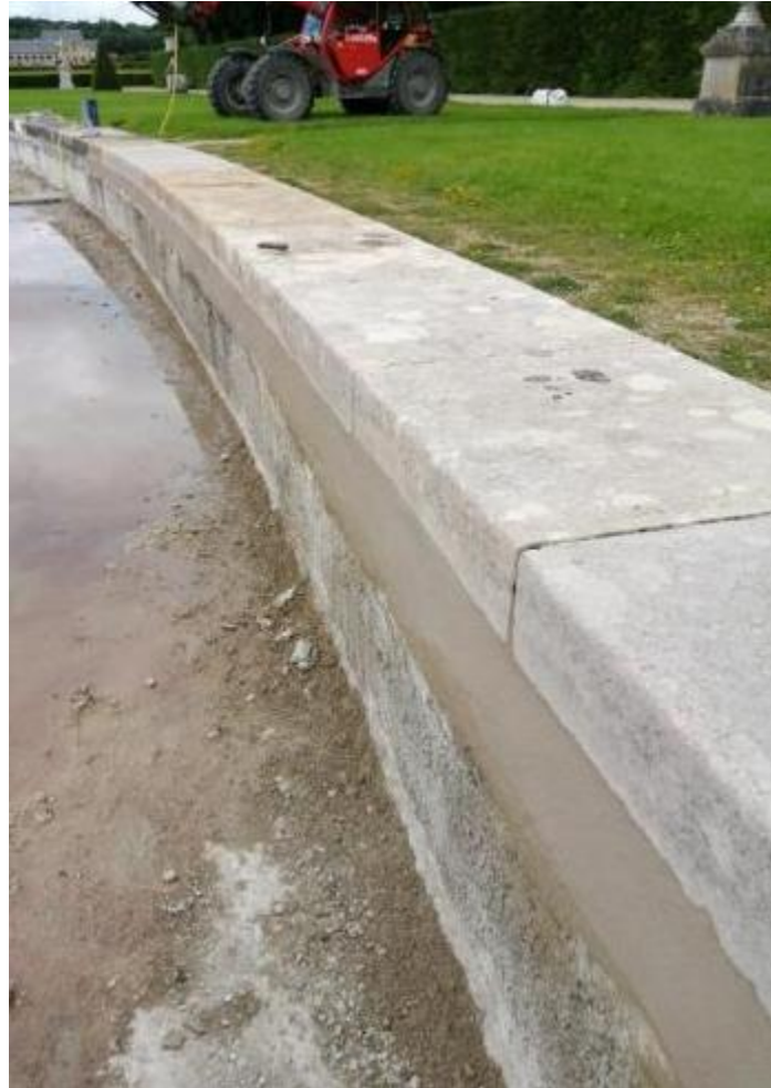
Repairing and waterproofing pools
