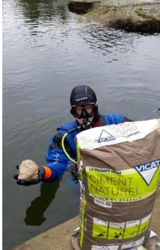
Sealing infiltration through dam masonry
