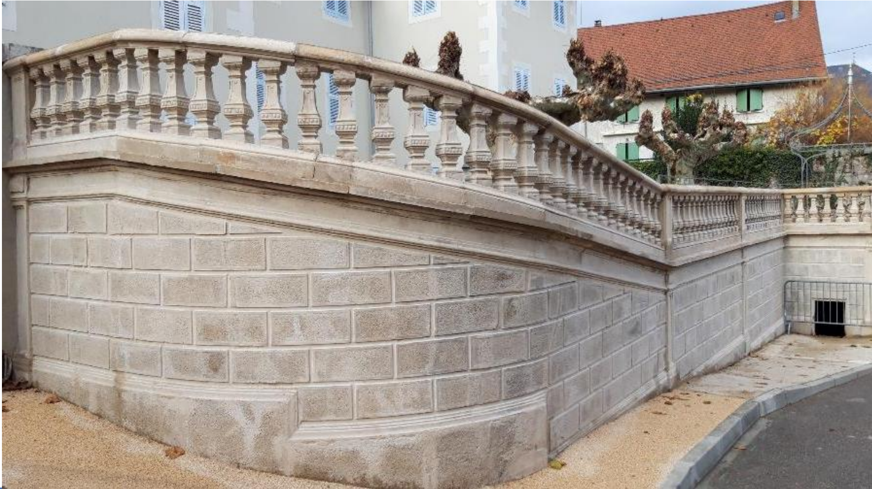
Moulding of balusters and artificial stones in Prompt natural cement concrete
