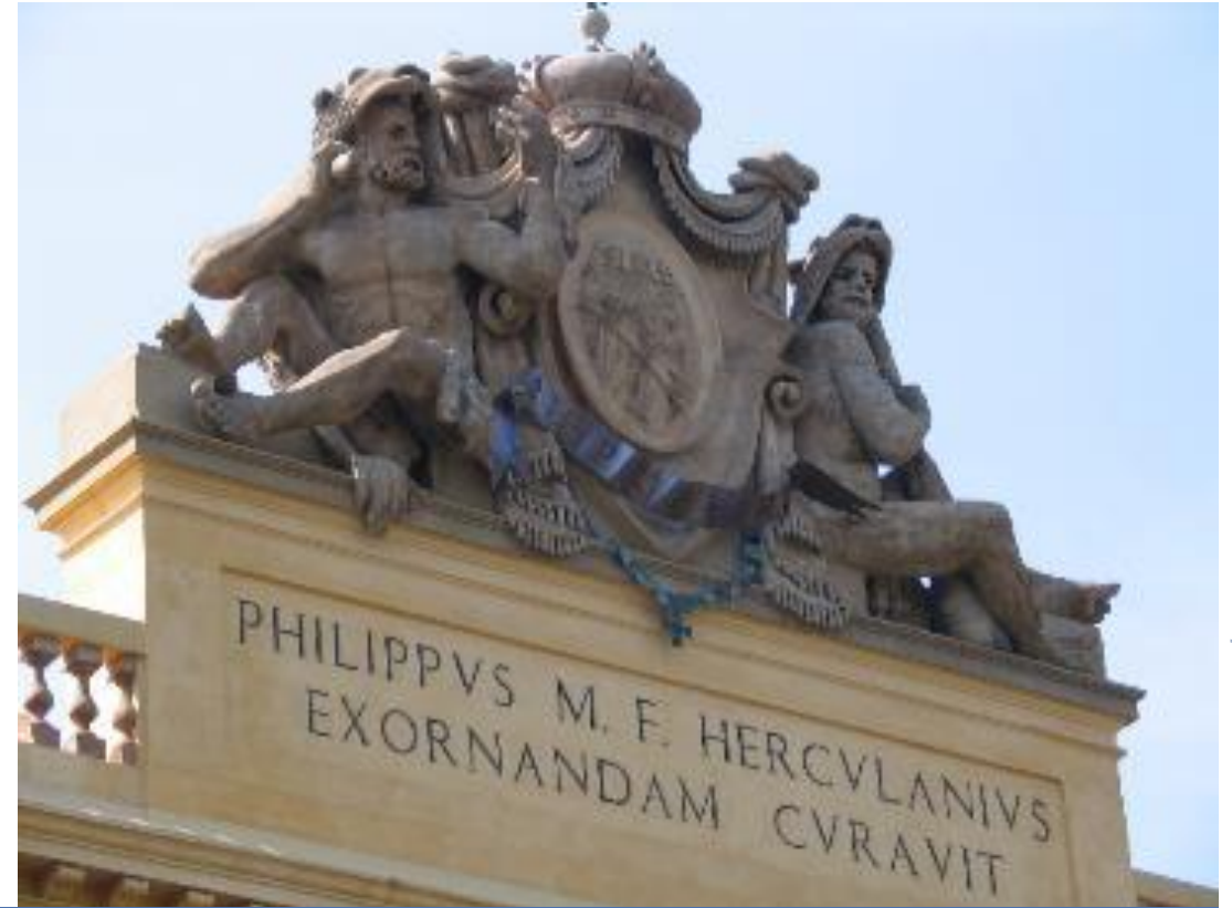
Restoration of statues and decorations in Prompt Natural Cement mortar
