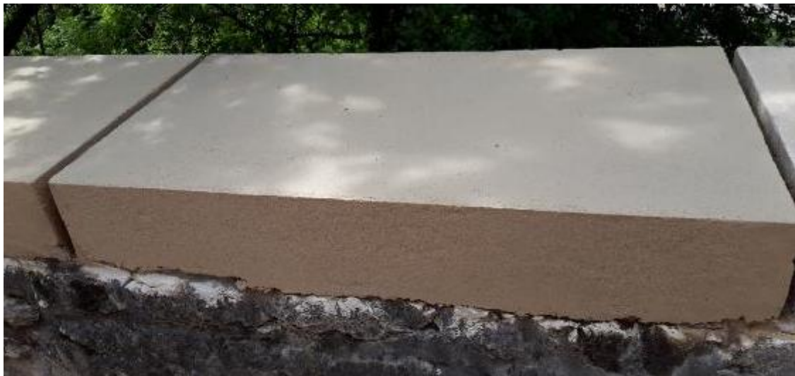
Replacement of the molasse stone covers with cast-in-place prompt concrete elements
