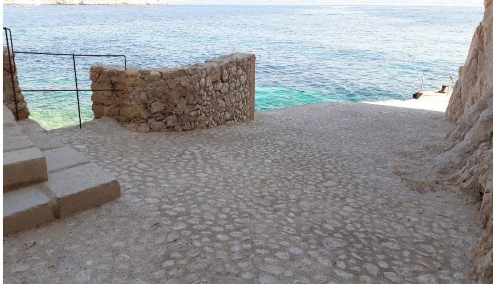
Paving on Lime/Prompt concrete base - Full joints
