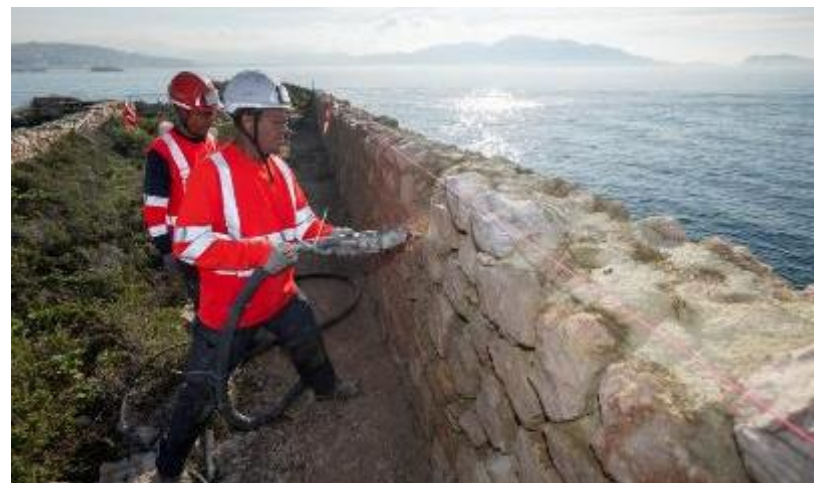
Repointing the walls by using lime / Prompt mechanical spraying mortar
