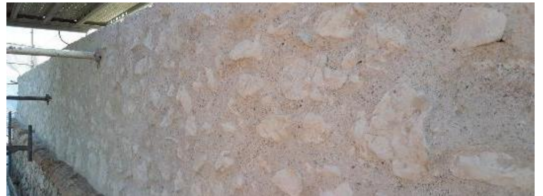
Repointing the walls by using lime / Prompt mechanical spraying mortar
