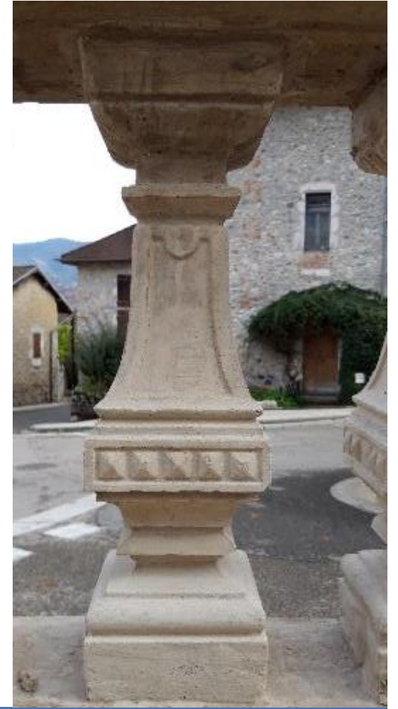
Moulding of balusters and artificial stones in Prompt natural cement concrete
