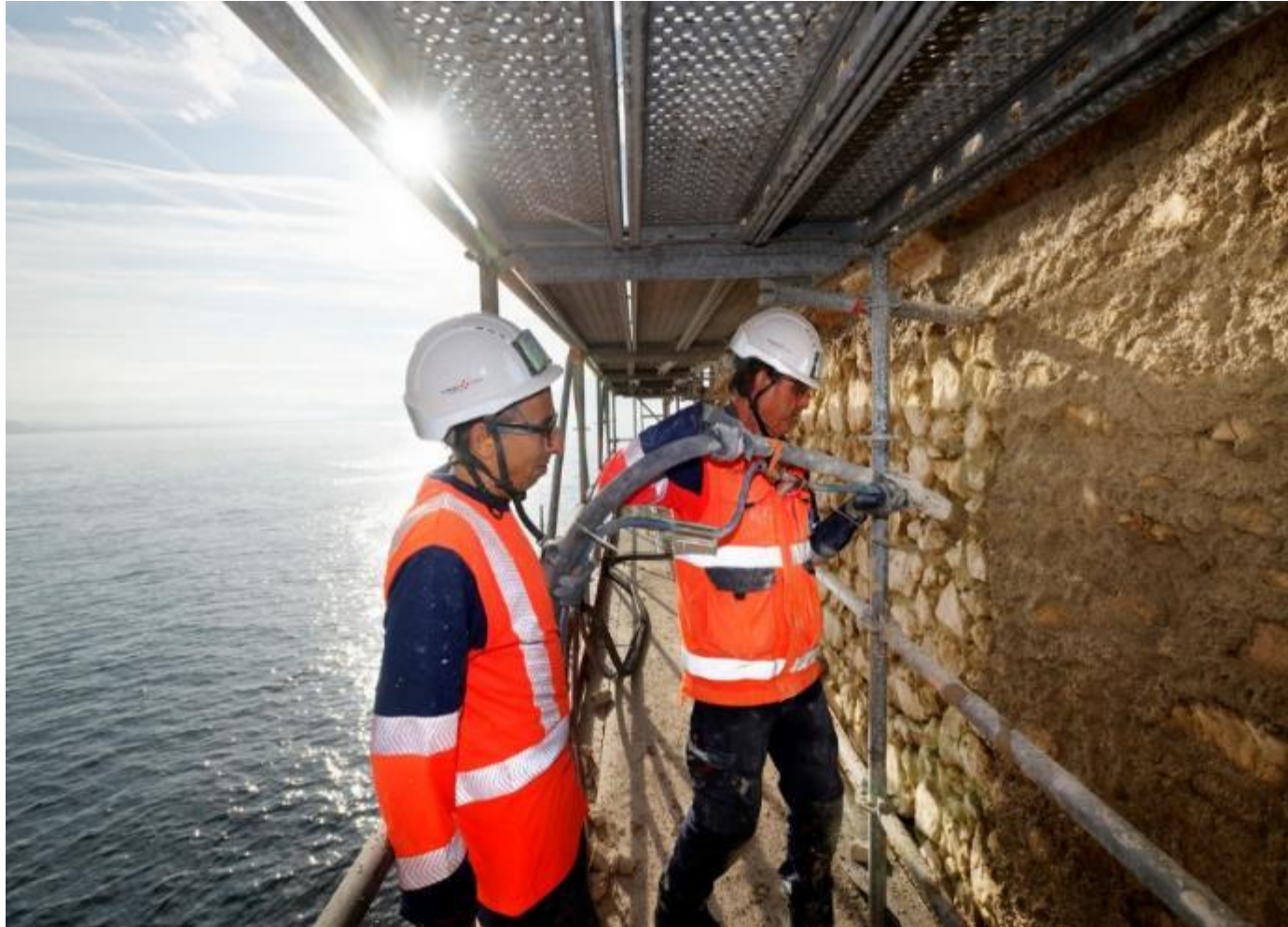
Repointing the walls by using lime / Prompt mechanical spraying mortar
