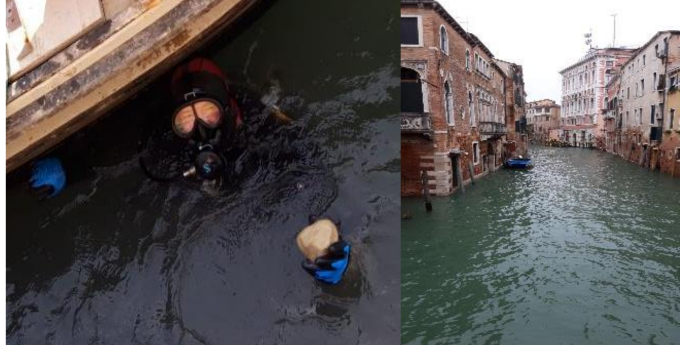
Prompt repair and sealing by a diver
